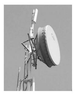
Figure 6.23 Photo of a parabolic reflector 'dish' antenna with shroud and radome.
